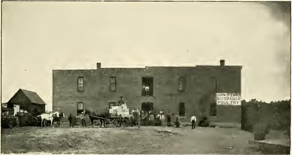
COMMISSION HOUSE OF JOHN STEWART, ONE OF CONCORDIA'S MOST EXTENSIVE INDUSTRIES.
